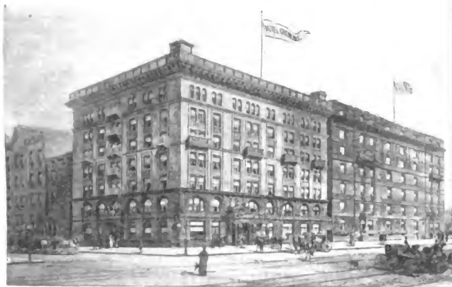
HOTEL GRENOBLE, SEVENTH AVENUE, FROM 56TH STREET TO 57TH STREET.
